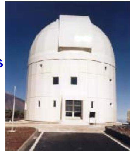
Optical Ground Station
